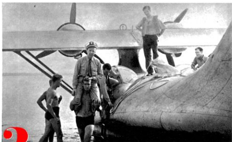
2 In large flying boats, another sea-anchor is attached by the ground-crew to aid in making this 90° turn. They also bring the pilots and air-crew members ashore from the Catalina pick-a-back to keep them dry.
